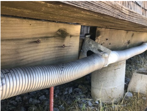
Center axle bracket twisting away from the wood
