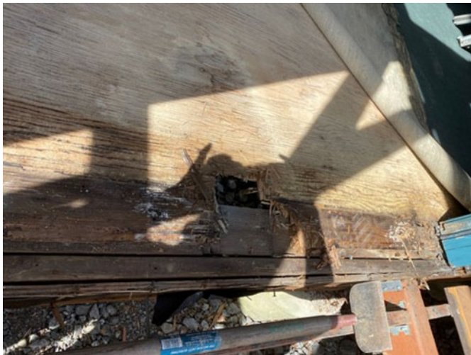
Double door "soft spot" and termite damage
