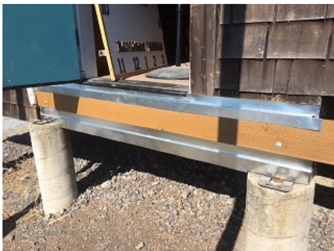
Repair of water damage under West door
